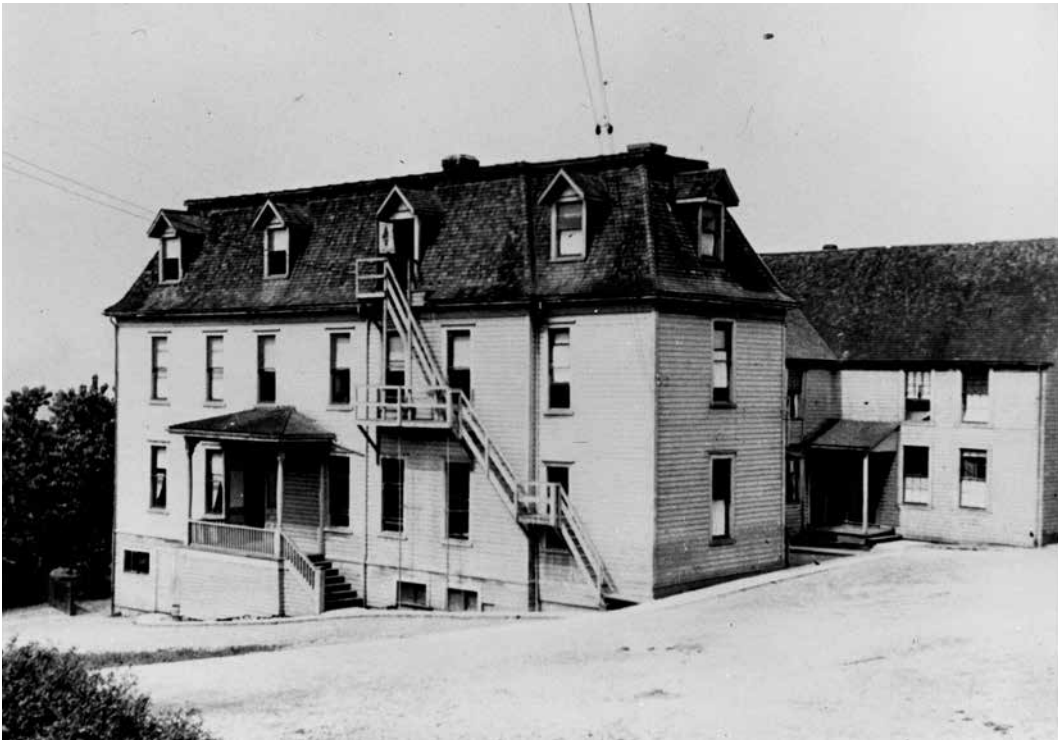
A 1958 inspection of the North Vancouver, British Columbia, school concluded that the school was "over crowded" and a "Fire Hazard." North Vancouver Fire Warden A. H. Abbott estimated that if the school caught fire at night, at least half the students would be lost. North Vancouver Archives, 4838.
